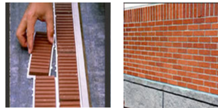
Figure 8.1 (left): Flat Brick Casting Figure 8.2 (right): Final Panel Look
